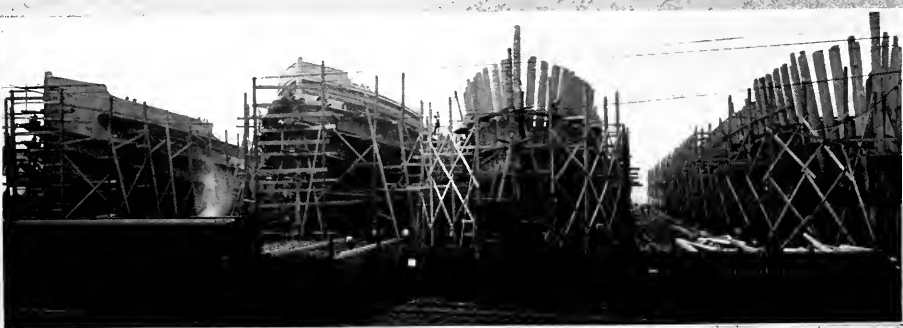
Four wooden steamers under way at the Supple and Ballin plant, Portland, Oregon. These vessels are built on the Ballin steel topsides principle and are extremely staunch and well fastened craft.
